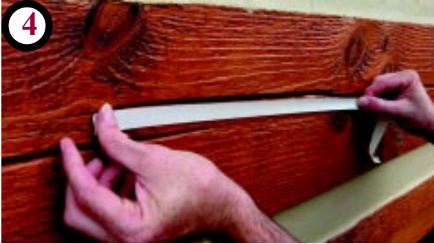
For neatest and cleanest job use masking tape above and below check
