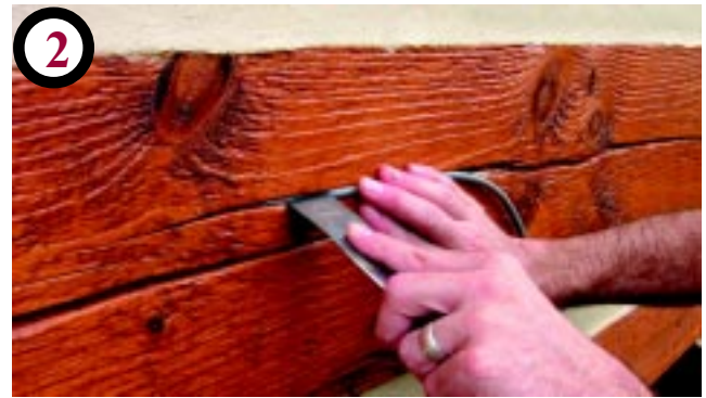
2 Fill check with appropriately sized Backer Rod
