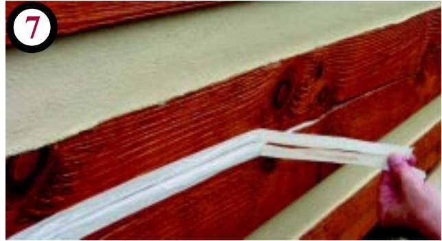
Remove masking tape while Check Mate is still wet
