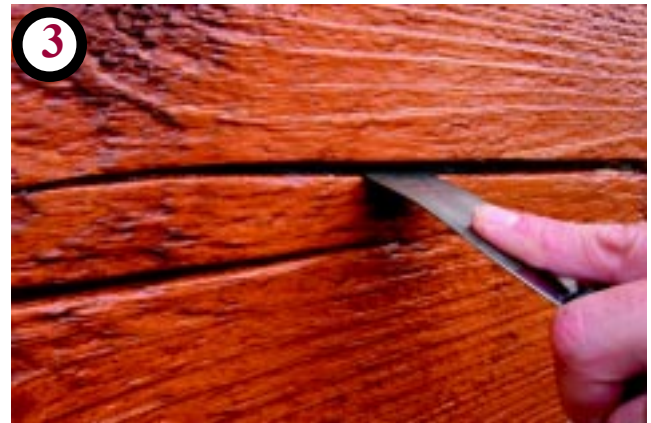
3 Push Backer Rod at least 1/4" into check
