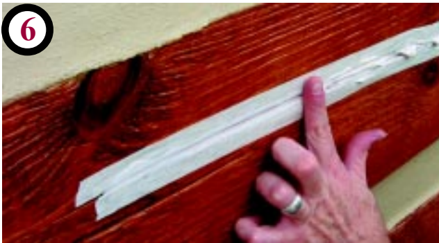
Smooth surface with a tool or wet finger
