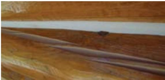
*Check-Mate 2 applied to upward facing check*
