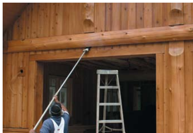
Application of Lifeline Advance clear topcoat over Lifeline Ultra-2 stain
