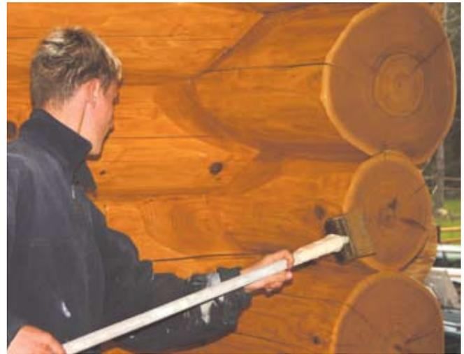
The exterior checks that face upward and could catch water should be sealed with *Check Mate 2* to prevent any further water entry. If the edges of the check are unprotected due to loss of finish, lightly sand the area and touch up with the appropriate color of finish and topcoat.
