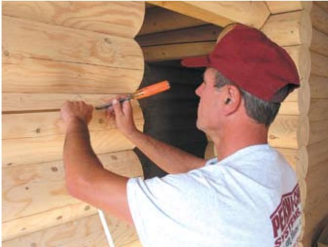
unfinished. The wicking problem can easily be cured by sanding the log ends to remove any old finish and caulk, as well as any surface deterioration that may be left. If there is moisture present in the ends, allow time for drying and then treat with *Shell-Guard RTU* wood preservative to stop any further progress of rot or decay fungi that may be present. When the *Shell-Guard RTU* has had time to dry, re-stain with the appropriate color.
