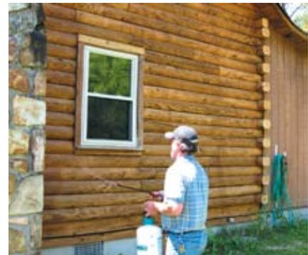
The borates are also recognized as being the most effective "green" wood preservatives that are available. The *Shell Guard®* is also very quick drying, and one application is normally all that is needed as long as the finish remains intact. Plus there is no "poison" smell and as it has no color, it removes the worries about it changing the color of your finish.
