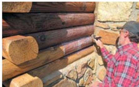
The application of *Prelude*<sup>™</sup> is much the same as the finish application; use an airless and spray until the point of run-off and back brush to work it into the fissures and checks on the logs as well as to brush out any runs. You can also use the “brush and bucket” method if you’re one of the traditionalist types. It dries fairly quickly and cleans up with soap and water.
