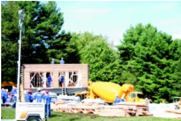
First wall being raised
