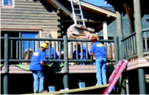
Volunteers applying Lifeline stain to the deck railings
