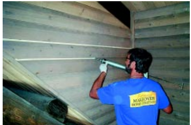
Keith Bedel from Northern Chinking in Maine applying Energy Seal
