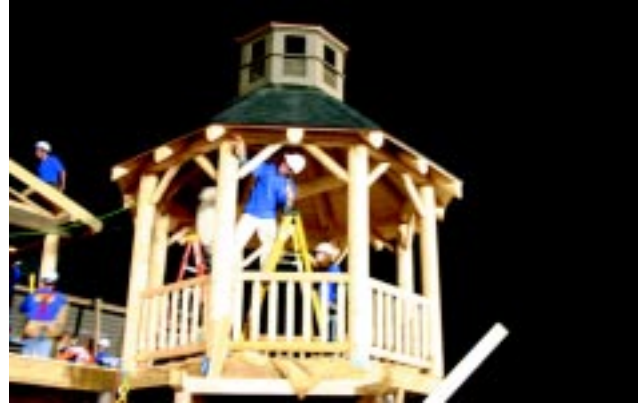
A crew from Lafontaine Painting, Vermont applying stains to the gazebo
