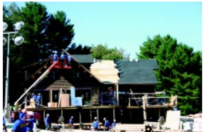
Man lifts were used for applying stain to the facia
